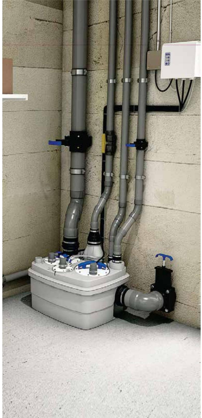
Saniflo offers a range of macerating and grinding pump systems that greatly reduce the size of fecal matter and waste. Larger diameter discharge lines are unnecessary; in fact, all that is needed is a 22mm diameter discharge line.
